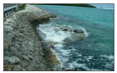
Figure 4.1-34. Coastal Erosion Protection along Route 11
